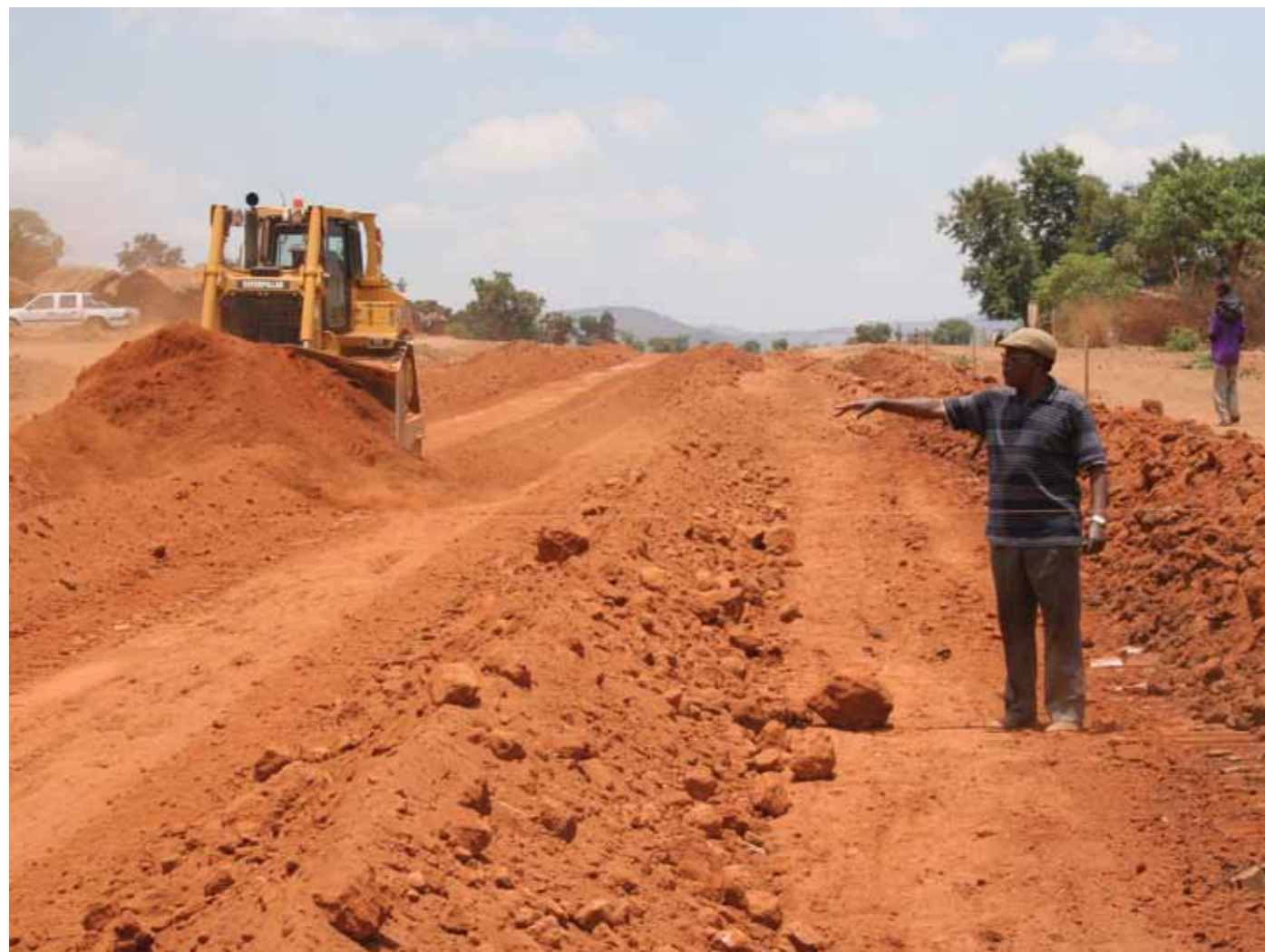
Works in progress on the Lumbadzi - Dowa road
