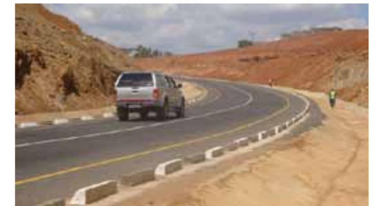
Different sections of the new Ekwendeni - Ezondweni road in Mzimba District
