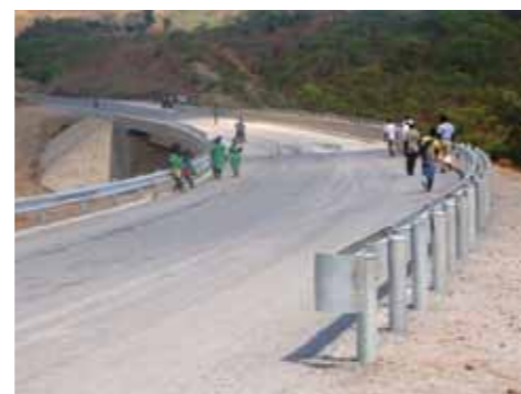
Four views of the construction of the newly completed Karonga - Chitipa road was completed in 2012
